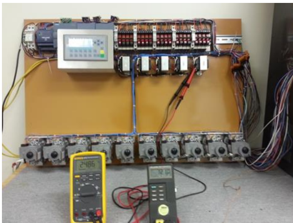
Far left: PLC power unit and power connections.
